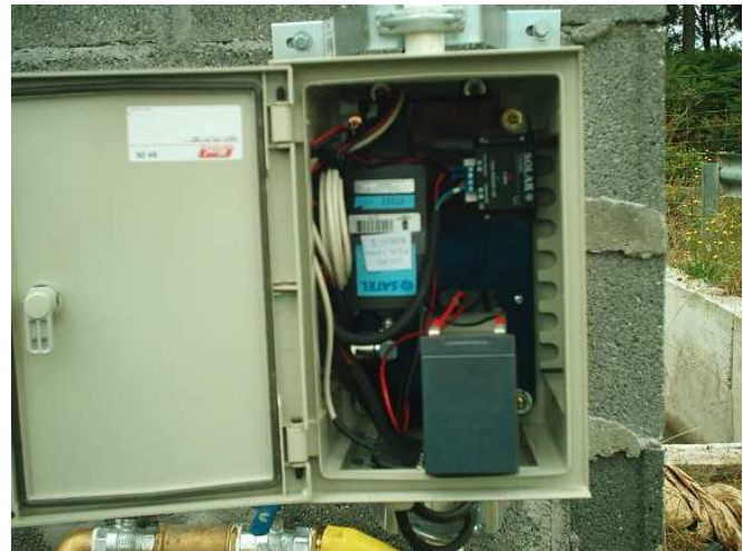
Figure 3: EZS data acquisition and communications system assembled in the protection box.
