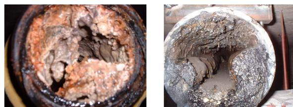
Figure 1 Scaling of the aged drain pipe
