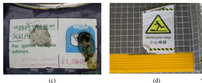
Fig.1. Examples of safety signs with different types of damage.
