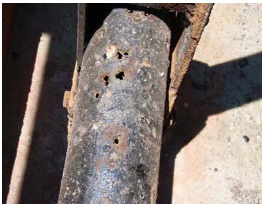
Fig. 2. Holes in the pipes.
