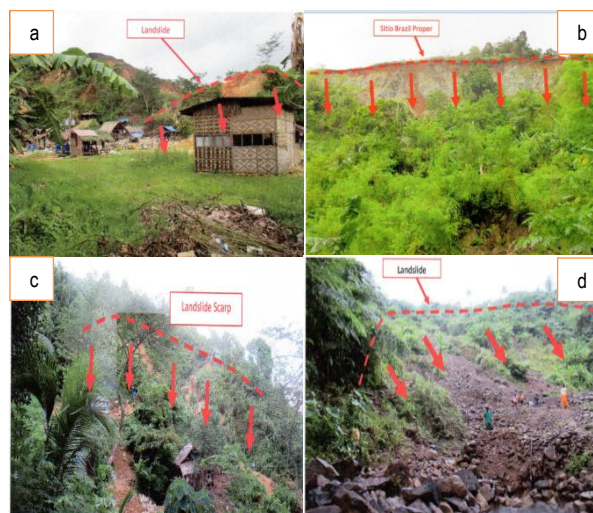
Fig 2. Panoramic view of some mining areas (a) GoldDustSlide1, Magsaysay, Placer; (b) BrazilSlide2, Sitio Brazil, Mat-i, Surigao City, (c) CansayongSlide2, Brgy. Cansayong, Malimono; (d) SanPedroSlide2, Brgy. San Pedro, Alegria
