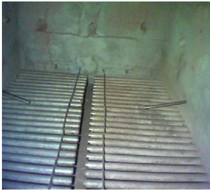
Fig 1. Sparge Pipe Distributor in a Fluidised Bed
