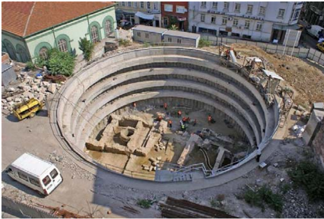
Figure 9: Sirkeci West Shaft Archaeological Excavations
