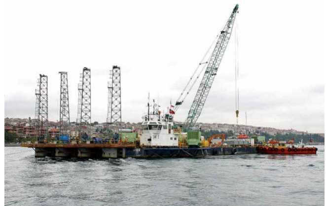
Figure 6: Compaction Grouting Works in the Istanbul Strait
