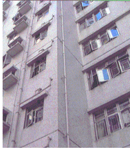
(b) Window is right-angle away from the gas pipe
