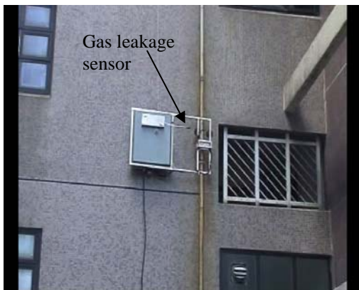
(e) It started automatic mode and tracked the gas pipe, and detect gas leakage from the installed gas leakage sensor.
