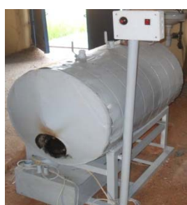
Fig 7: Side view of the Boiler
