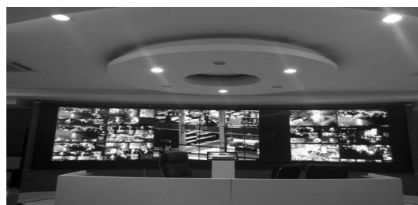
Figure 6. Municipal Condition from city CCTV monitoring.
