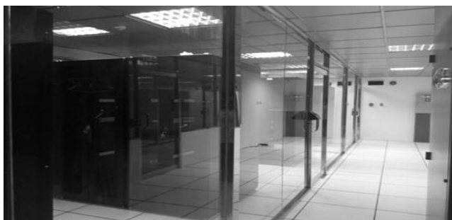
Figure 4. Data Centre 12 racks
