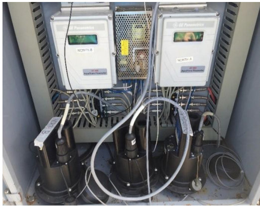
Fig. 5. A 3-channel Cello logger is installed to log the measured temperature by the thermocouple
