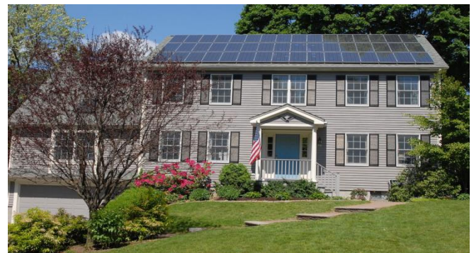
Fig .1 Photovoltaic array in houses
