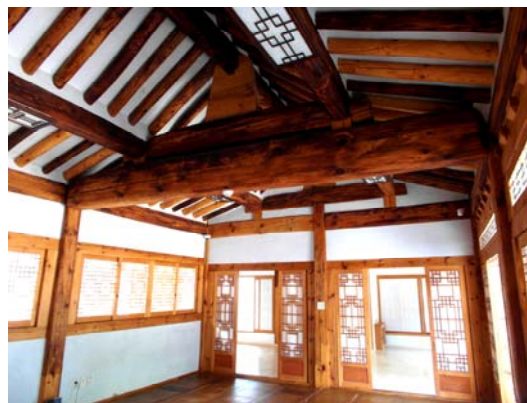
(b) Post and beam structure of traditional Hanok
