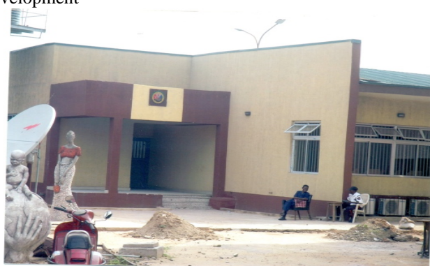
Fig. 5. Just Completed multimillion Naira Computer Laboratory for Practical computer Training for students and Staff
