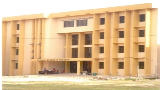
Fig. 2. Just completed new school of Science with several classrooms, laboratory and staff offices
