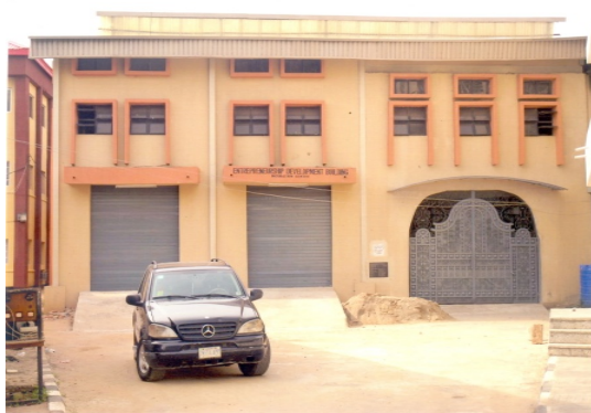
Fig. 4. Completed EDP center, where students acquire knowledge practical knowledge on entrepreneurship development
