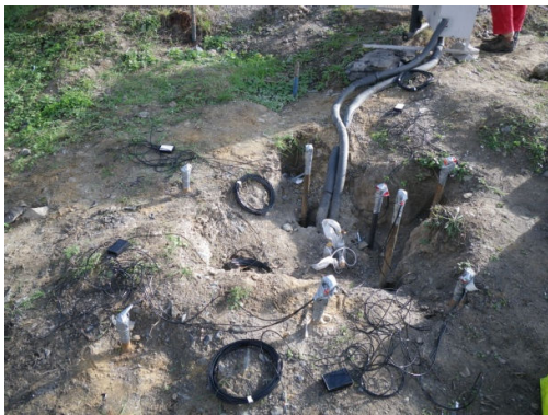
Fig. 5. Installation of measurement system around the heat collector
