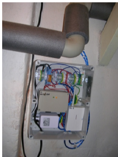
Fig. 4. Overview of installed evaluation unit
