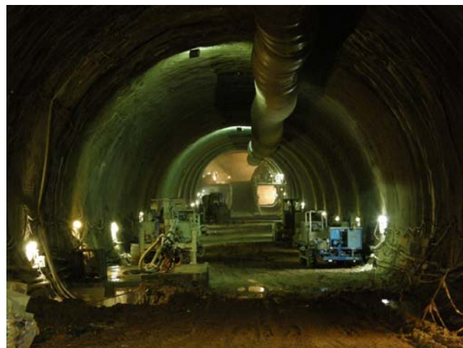
Fig. 1. A view of drilling in the tunnel
