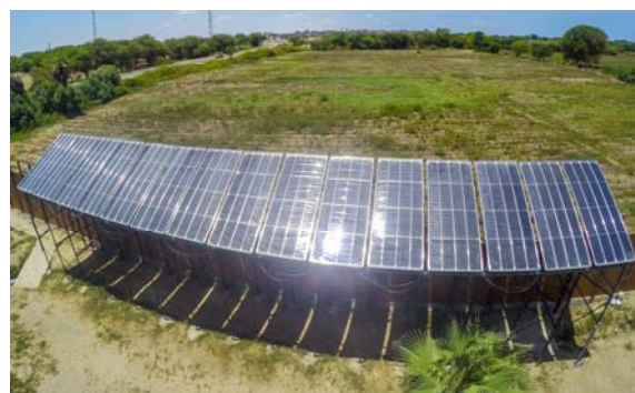
Figure 2.- Distilling panels installed
