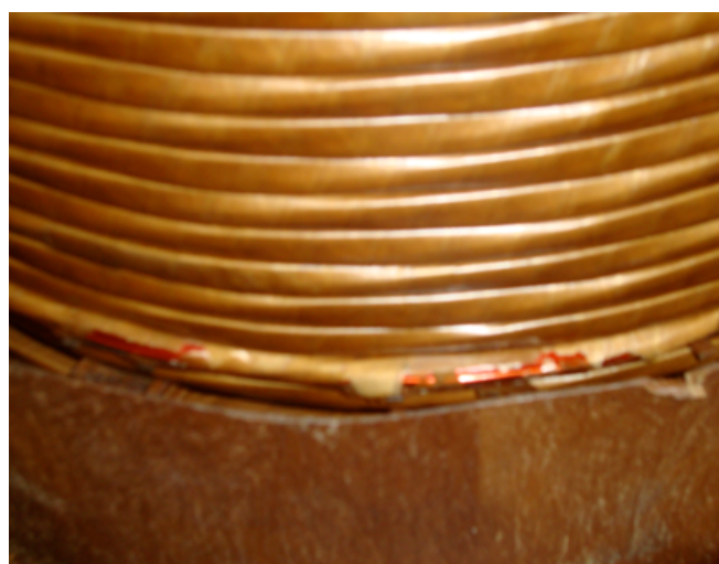
Fig. 11. Phase B winding inspection
