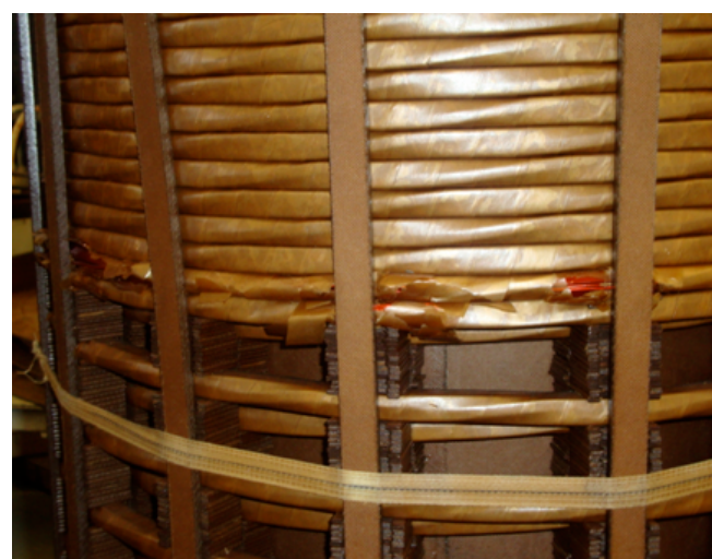
Fig. 8. Phase C low voltage winding
