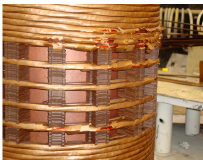
Fig. 9. Phase C low voltage winding
