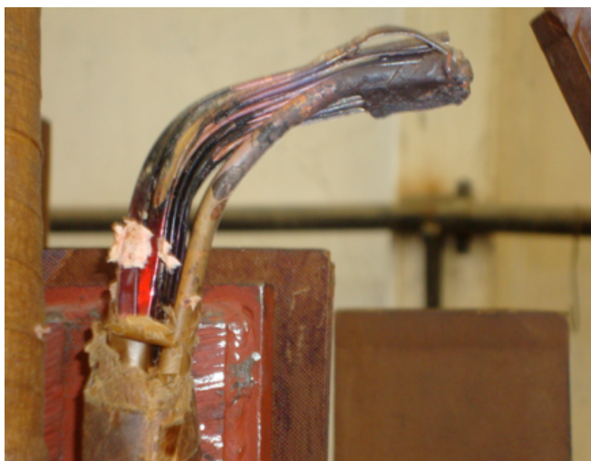
Fig. 4. Phase B conductor damage
