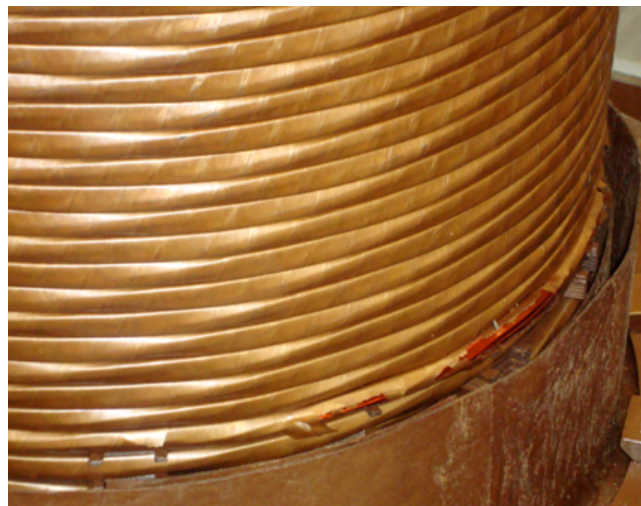
Fig. 10. Phase B winding inspection
