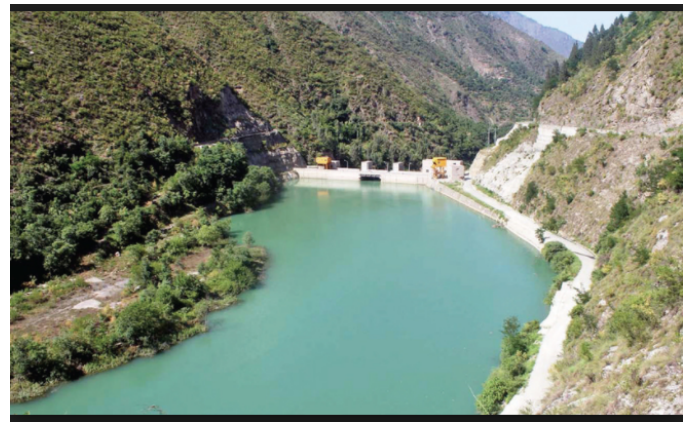
Fig. 1. KKHPP dam view from upstream
