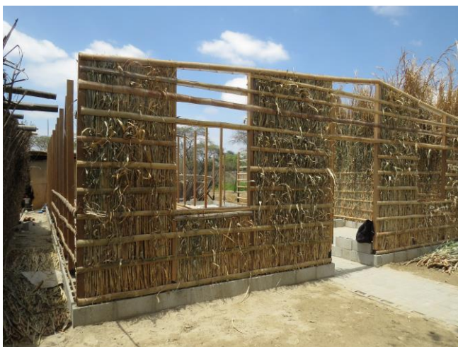
Fig. 7. Materials of the house.
