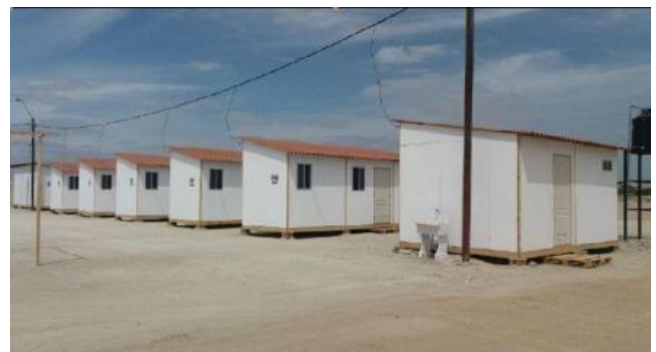
Fig. 2. Initial Housing Unit
