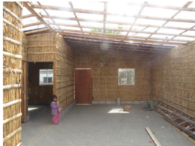
Fig. 5. The ventilation of the house is due to the roofs high and walls material.
