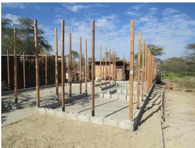
Fig. 8. Solid Structure of the house base.
