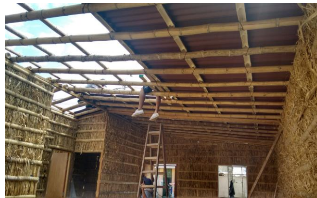
Fig. 4. Implementation of the post-disaster housing roof.
