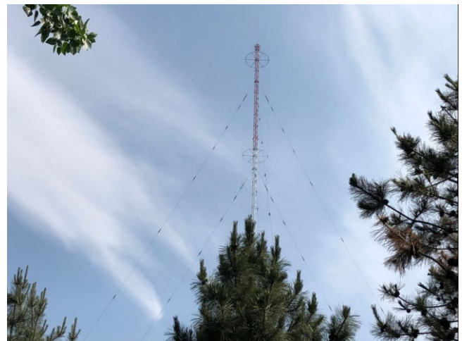
Fig. 16. Photograph of a 200 kW medium-wave 639 kHz antenna in Fangshan District, Beijing for broadcasting radio signals over long distances.
