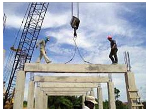
Fig.1. Assembling of Precast concrete element
