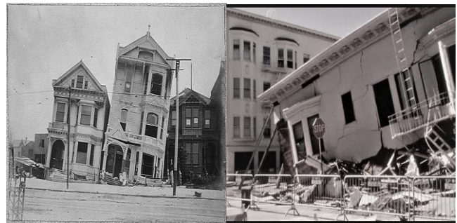
Fig.1. Example of Punching Shear failure in the buildings due to earthquake.
