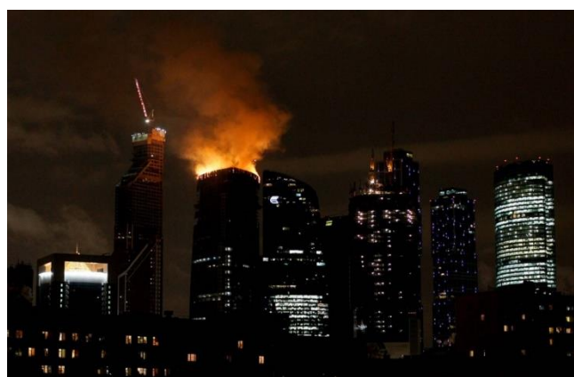
Fig.1 Fire in Tower East (The Federation Towers), 02.04.2012 (from supercoolpics.com).
