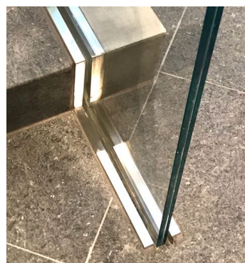
Fig. 16. First floor glass guardrail, as it starts, anchored into the lobby floor, prior to the first riser step rising up the angled monumental three-story staircase. Note the plastic laminate internal strip is visible.
