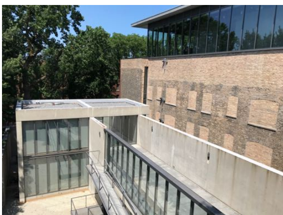
Fig. 18. Exterior view looking north, from roof of owner’s home towards northwest corner of Wrightwood 659 gallery building. Note filled-in window openings of former apartment building, along with new fourth-level of gallery building, being clad in floor-to-ceiling reflective glazing.
