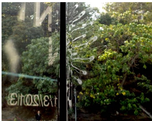
Fig. 9. Dendritic patterns of air intrusion in failed laminated glass panels. Asia Society building in Admiralty district, Hong Kong, S.A.R. China. Condition observed on site by author, 24 February, 2013.
