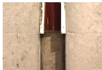
Fig. 13. Interior elevation of vertical embedded 'groove' in architectural finish Ando concrete wall; horizontal joint line subtly stretches across center of image. Dark maroon FinnForm formwork with white epoxy-adhered edge banding is visible; lower portion of formwork has been removed prior to taking this on-site photograph on 5 December 2017.
