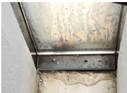
Fig. 1. Condensation upon narrow slit window at Pulitzer Arts Foundation, Observed February 2015.
