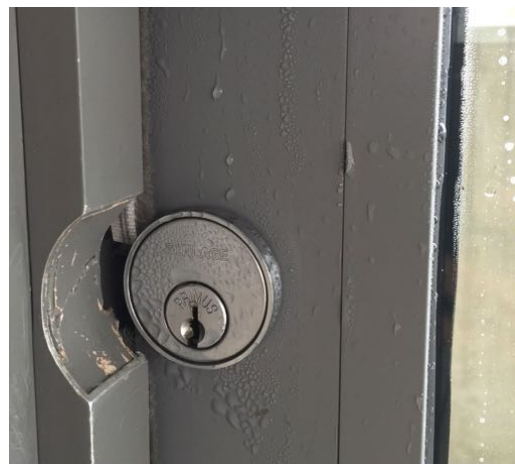
Fig. 2. Condensation upon door side stile and lockset at Pulitzer Arts Foundation, Observed February 2015.
