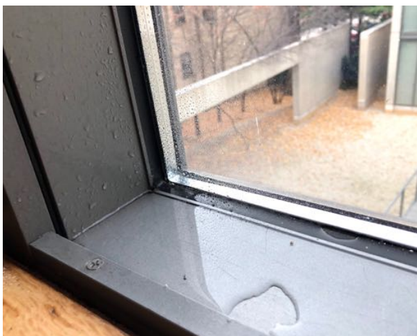
Fig. 3. Condensation upon non thermally broken aluminum sill of combination door and operable window, Wrightwood 665 Private Residence, Chicago, Observed Winter 2014.
