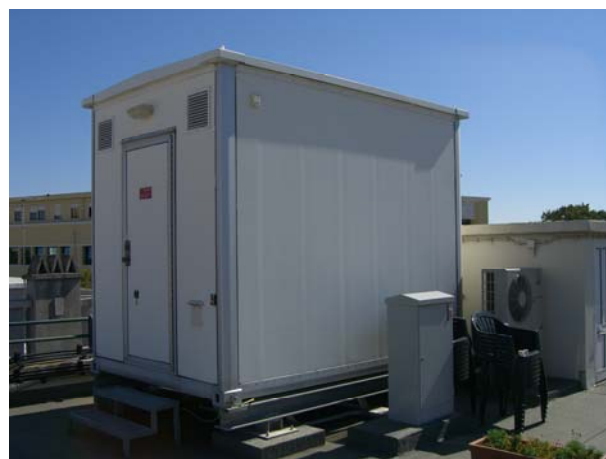
Fig. 1 – Photograph of the exterior of one of Vodafone's base stations.
