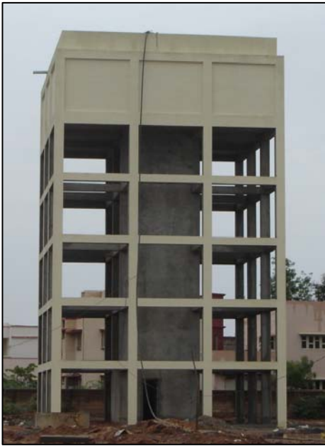
Fig.2. Image of selected ESR located at Bhuj, Gujarat
