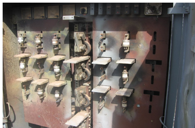
Fig-7: Copper links used as Fuses
