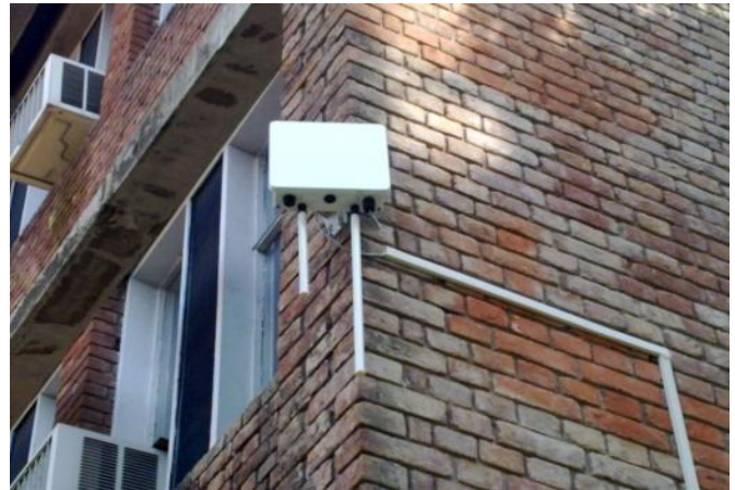
Fig. 3(a): wireless mesh portal connected through Ethernet
