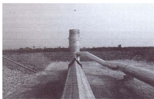
Fig. 3: Flare Stack with AISI 446 SS Burner ready for Service.
