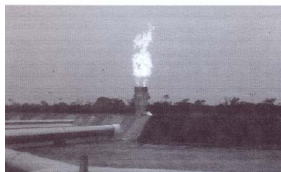
Fig. 4: Flare Stack with AISI 347 SS Burner in Service.
