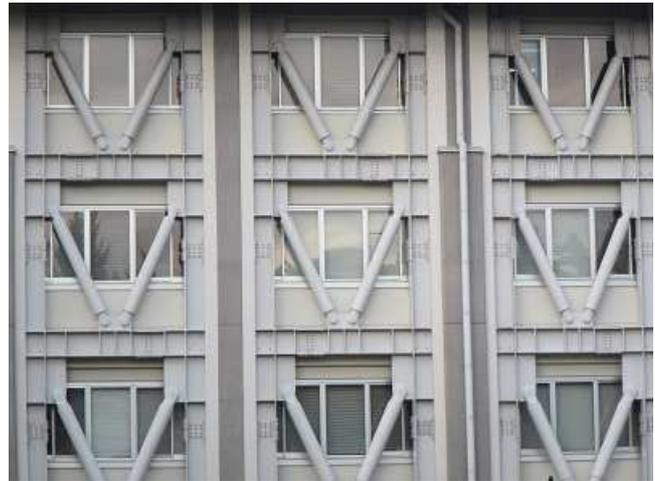
Fig. 1. Earthquake-Resistant Dumpers for building.
