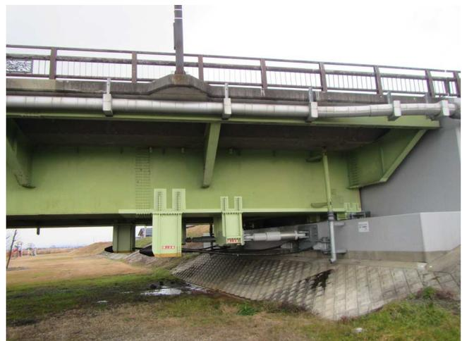
Fig. 2. Earthquake-Resistant Dumpers for bridge.
