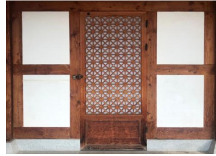
Fig. 2. Hanok styled shear wall. Shear wall consists of soil wall with horizontal intermediate member called Inbang and has door opening.
