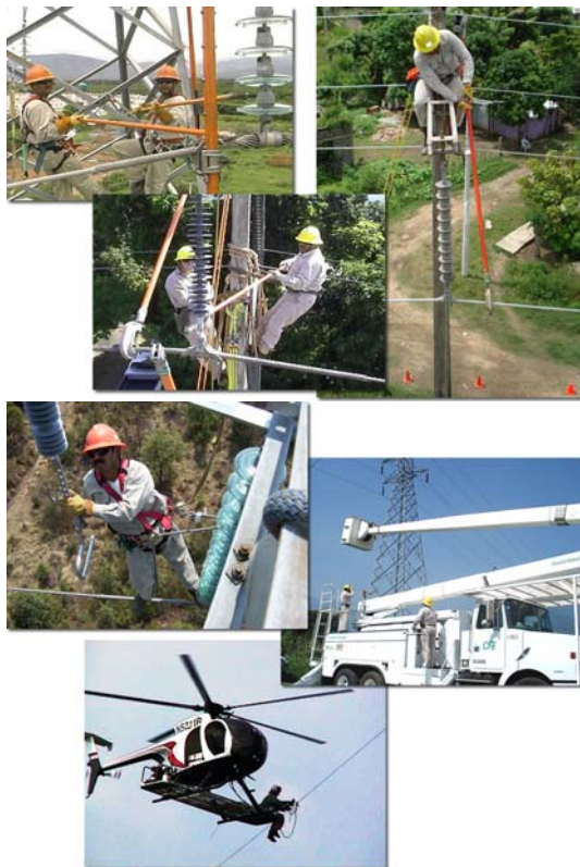
Figure 1. Some examples of maneuvers for live-line maintenance.
